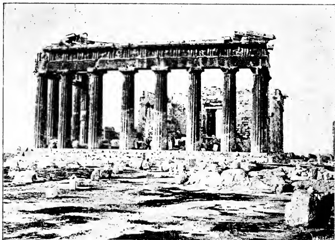
FIG. 60.—PARTHENON, FROM THE EAST.
